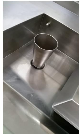
Cup sink (perforated cover removed)
